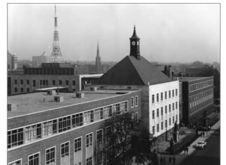
FIG. 7. GENERAL VIEW OF SOUTH ELEVATION, KERR HALL CIRCA 1964. | COURTESY OF RYERSON UNIVERSITY ARCHIVES, DOC FL: HOWARD KERR HALL.
