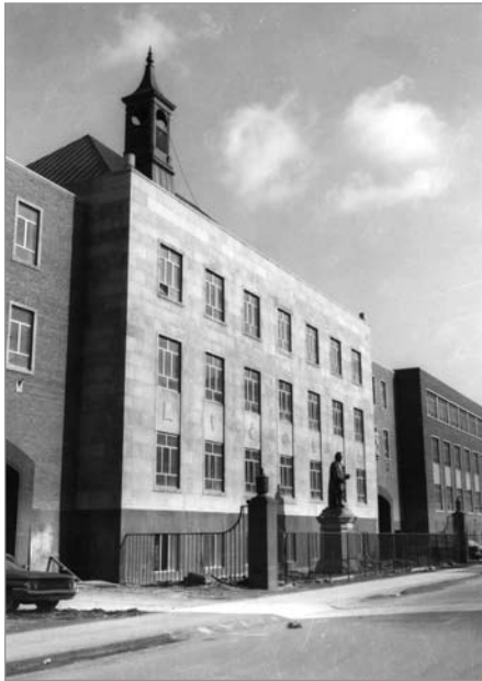
FIG. 9. KERR HALL, CIRCA 1961, SOUTH FAÇADE ON GOULD STREET. | COURTESY OF RYERSON UNIVERSITY ARCHIVES, DOC FL: HOWARD KERR HALL.
