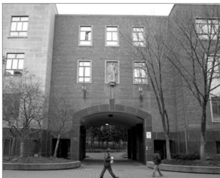
FIG. 10. KERR HALL, LINK WITH PASSAGE TO COURTYARD FROM GOULD STREET. | MARYBETH McTEAGUE.
