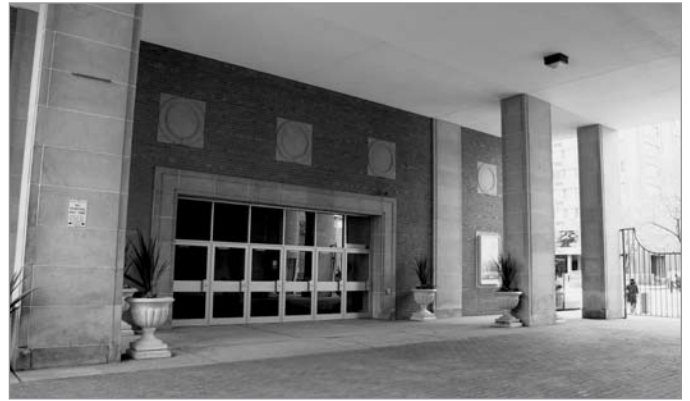
FIG. 16. THEATRE ENTRANCE, KERR HALL, NORTH PASSAGEWAY TO GERRARD STREET. | MARYBETH McTEAGUE.
