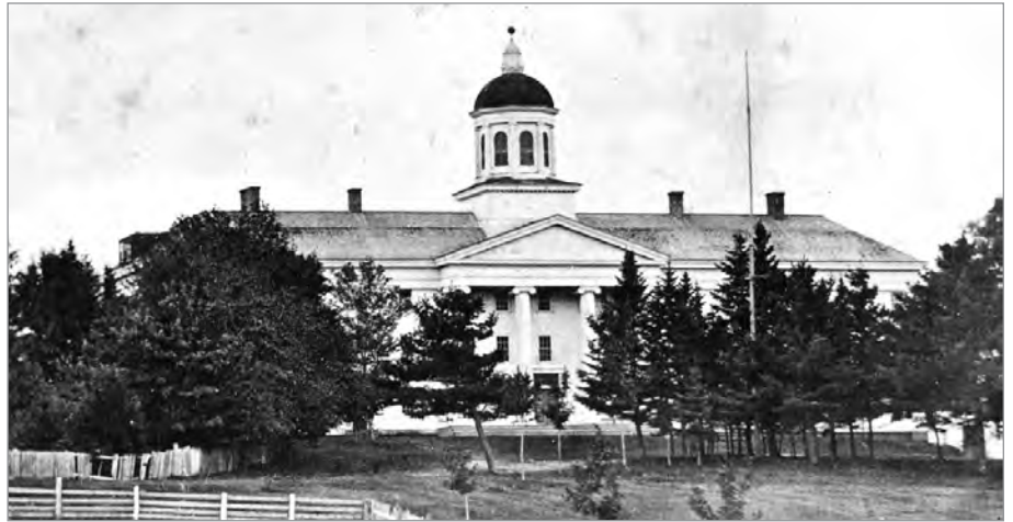
FIG. 6. FIRST COLLEGE HALL, ACADIA COLLEGE, WOLFVILLE, C. 1880. BURNED 1887. | ESTHER CLARK WRIGHT ARCHIVES, ACADIA UNIVERSITY, APC968.
