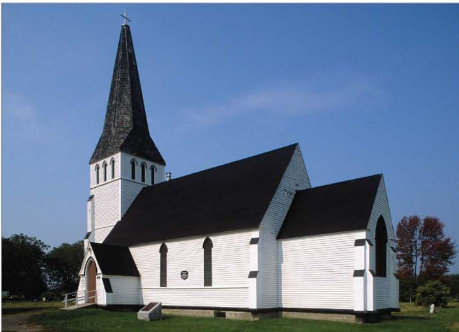
FIG. 1. CHRIST CHURCH, MAUGERVILLE (NB), EXTERIOR FROM SOUTHEAST. | MALCOLM THURLBY.
