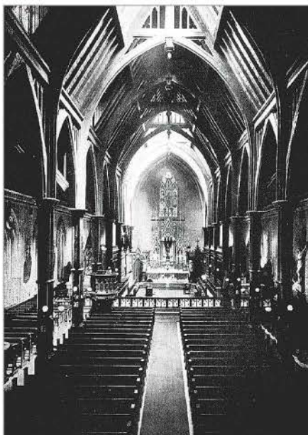
FIG. 16. ST. BASIL'S CATHOLIC CHURCH, TORONTO, ARCHIVAL PHOTOGRAPH – INTERIOR LOOKING EAST. | COURTESY OF THE UNIVERSITY OF ST. MICHAEL'S COLLEGE ARCHIVES.
