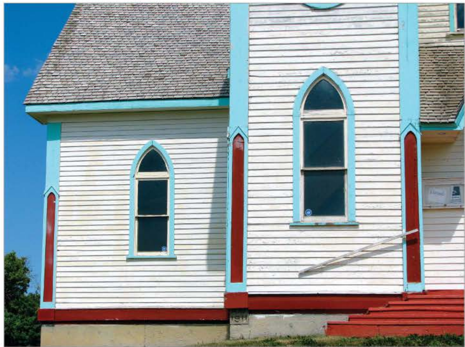
FIG. 15. DETAIL OF GABLETS MIMICKING MASONRY BUTTRESSES, BEKEVAR PRESBYTERIAN CHURCH, BEKEVAR, RM 94. | KRISTIE DUBÉ.
