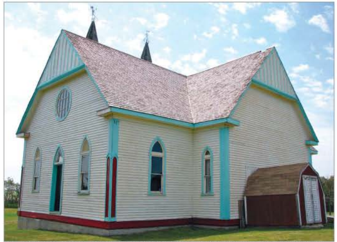
FIG. 11. VIEW OF THE SOUTHWEST PORTION SHOWING LANCET WINDOWS AND DELINEATED CHANCEL, BEKEVAR PRESBYTERIAN CHURCH, BEKEVAR, RM 94. | KRISTIE DUBÉ.
