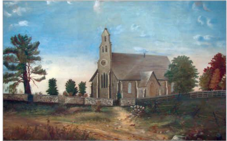
FIG. 33. ST. PETER'S ANGLICAN CHURCH (1852), BARTON, ANONYMOUS PAINTING NOW IN THE HALL OF ST. PAUL'S ANGLICAN CHURCH, GLANFORD (ON). | PAUL CHRISTIANSON, 2012.
