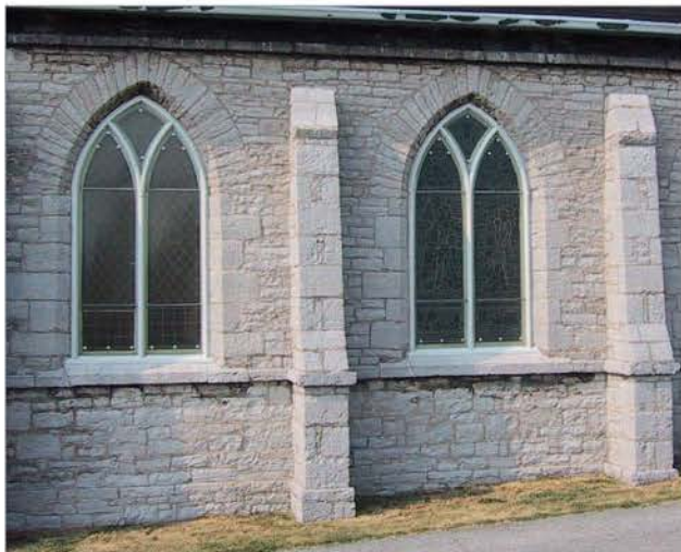
FIG. 8. ST. MARK'S ANGLICAN CHURCH, BARRIEFIELD, DETAIL OF STONEMWORK ON THE SOUTH FAÇADE. | PAUL CHRISTIANSON, 2008.
