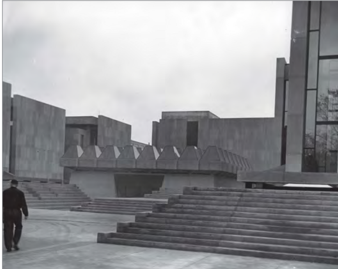
FIG. 2. THE CONFEDERATION CENTRE FOR THE ARTS WAS A PROTO-CENTENNIAL PROJECT COMMEMORATING THE CHARLOTTETOWN CONFERENCE. ALSO DESIGNED BY ARCOP, IT IS INTERESTING TO SEE THE FOCUS ON THE SCULPTURAL QUALITIES OF THE COURTYARD BETWEEN THE BUILDINGS, AND THE SIMPLICITY OF THE BUILDINGS THEMSELVES. | CANADIAN ARCHITECT MAGAZINE IMAGE COLLECTION, RYERSON UNIVERSITY.
