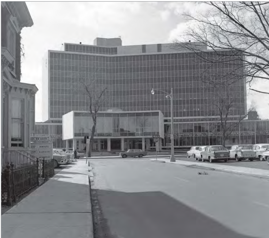
FIG. 1. VIEW OF HAMILTON CITY HALL IN THE CONTEXT OF THE VICTORIAN CITY, 1961. | RYERSON UNIVERSITY LIBRARY ARCHIVES AND SPECIAL COLLECTIONS.
