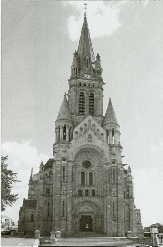
FIG. 11. SAINT-MARTIN'S CHURCH, VITRÉ, BUILT IN 1883 TO THE PLANS OF ARCHITECT HENRI MELLET, VIEW OF WESTWORK. | LUC NOPPEN
