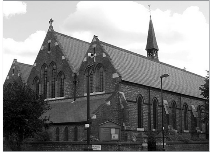
FIG. 18. ST. THOMAS CHURCH, ISLINGTON (LONDON), 1888-1889, EWAN CHRISTIAN. | [HTTP://EN.WIKIPEDIA.ORG/WIKI/FILE:ST_THOMAS%27S_CHURCH,_ISLINGTON.JPG] , RETRIEVED JANUARY 8, 2014.
