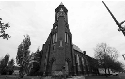
FIG. 22. NEW ST. PAUL'S ANGLICAN CHURCH, VIEW OF THE SOUTHWEST EXTERIOR. | LORYSSA QUATTROCIOCCI, NOVEMBER 21, 2014.
