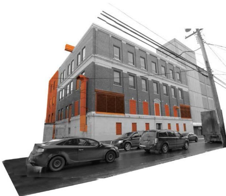
Image 07: Photograph of North Street Data Center taken from North Street at Agricola Street. Items highlighted in orange show the bricked over windows, mechanical upgrades and architectural additions to the building. Halifax, Nova Scotia, 2014.
