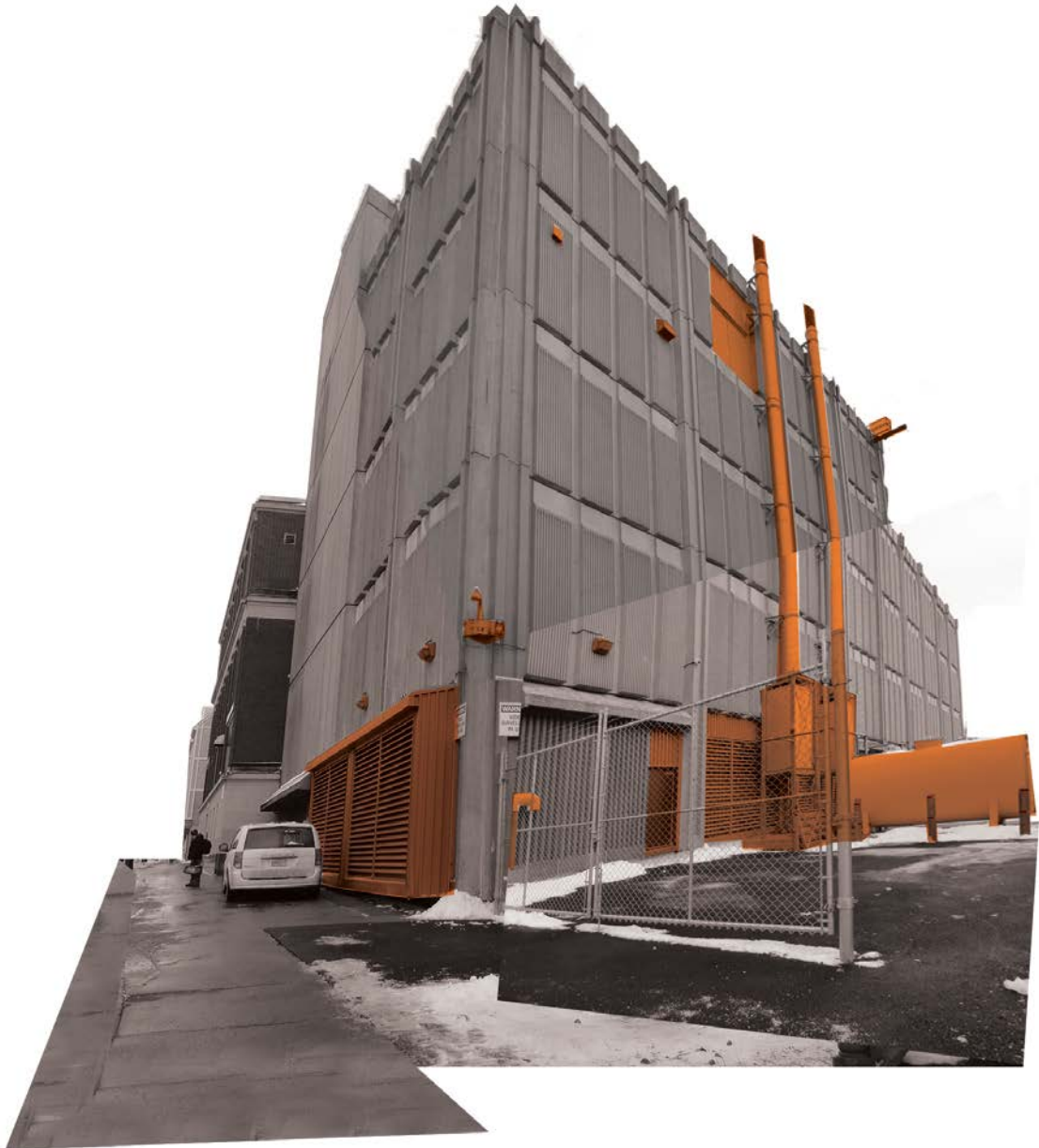
Image 09: Photograph of North Street Data Center taken from North Street at Robie Street. Items highlighted in orange show the bricked over windows, mechanical upgrades and architectural additions to the building Halifax, Nova Scotia, 2014.
