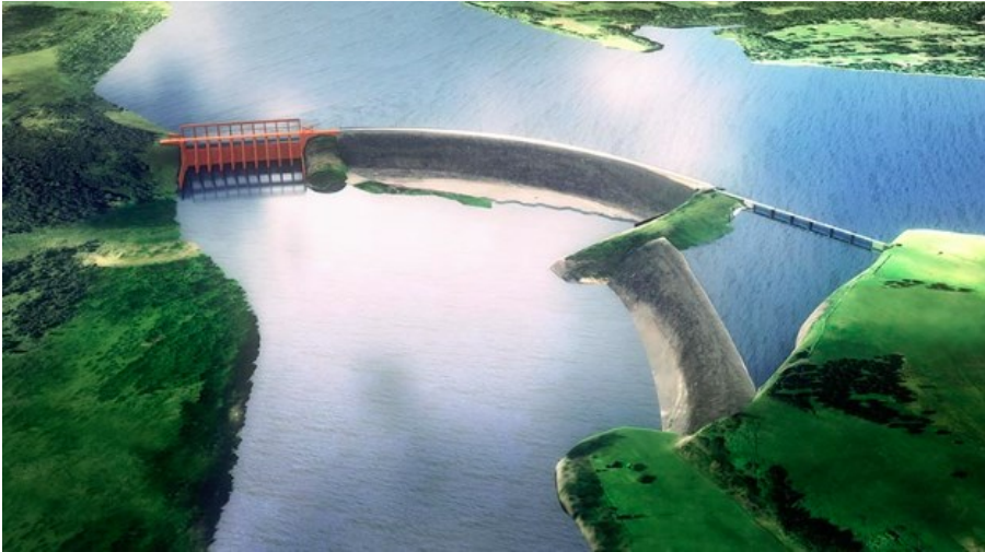
b. Visualization of option 2, retaining the headpond (no power), only the earthen dam is maintained
