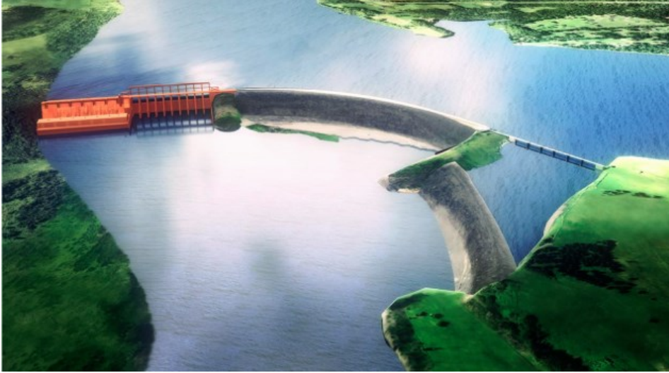
a. Visualization of option 1, repowering the dam, by rebuilding the spillway and powerhouse.
