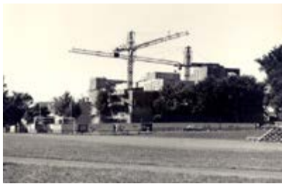
Life Sciences Centre - Under Construction - Construction Cranes, November 25, 1970
