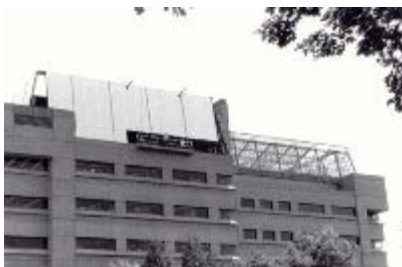
New 8th floor addition to LSC, July 1991
