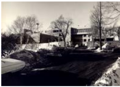
Construction Shot - Life Sciences Centre, 1971
