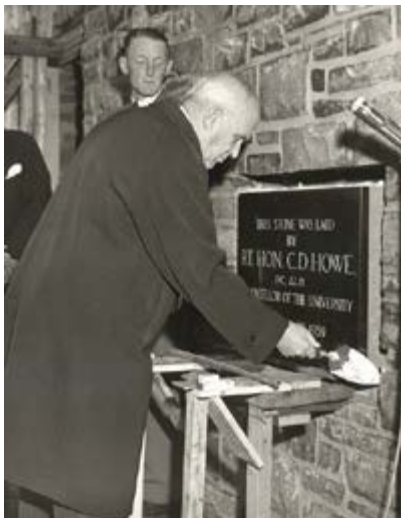
Cornerstone Laying - Men's Residence - Howe Hall, October 1959
