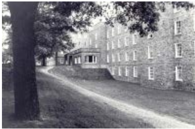
Howe Hall - Exterior, n.d.
