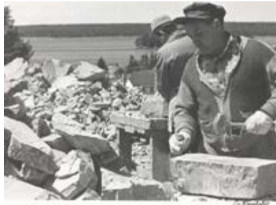
Men's Residence - Construction, 1959
