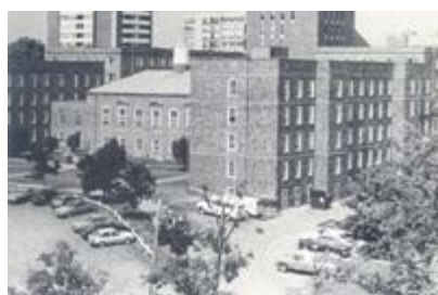
Howe Hall looking northeast, 1985
