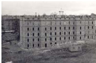
Howe Hall Men's Residence Under Construction, December 14, 1959
