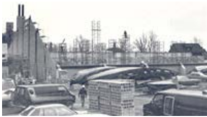
New rink under construction, 1981
