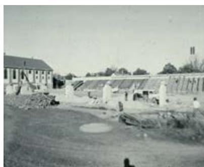
New Dalhousie Rink - Construction, 1981
