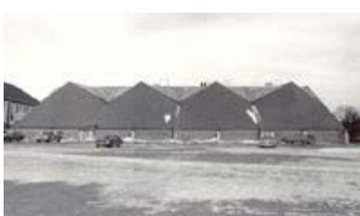
Dal Rink under construction, February 1982
