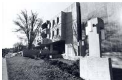
Arts Centre - Exterior - Front, 1975
