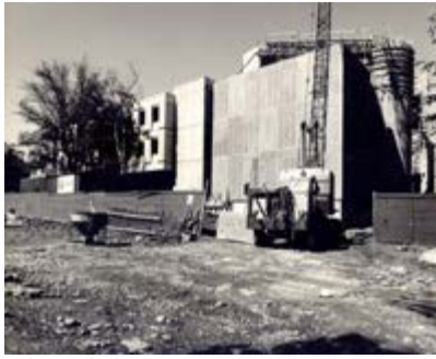
Arts Centre - Under Construction, 1970
