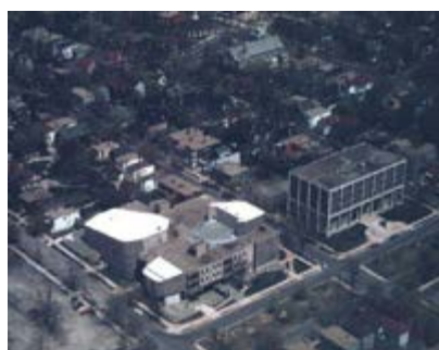
Aerial view of the Arts Centre, 1977
