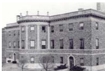
Chase Building - Exterior - Front - Angle View, February 25, 1980
