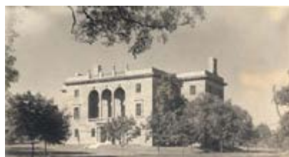
Chase Building - Exterior - Rear, n.d.
