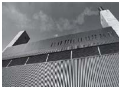
Central Services Building (formerly Physical Plant), c1970s
