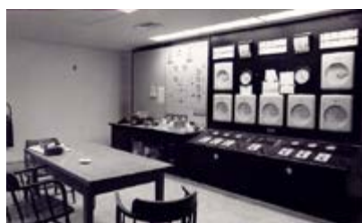
Central Services Building - Control Room, 1971
