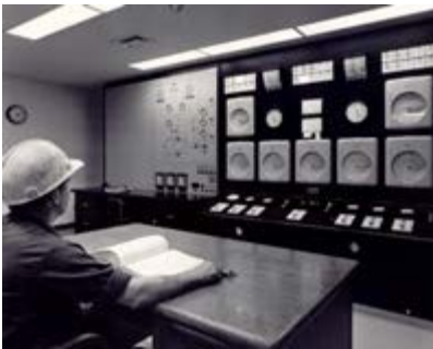
Control Room - Central Services Building, 1971
