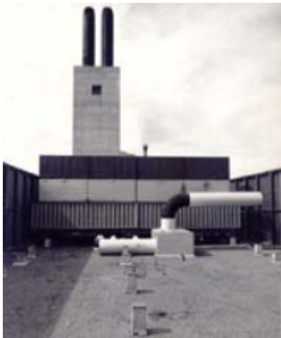
Central Services Building - Smokestacks, September 14, 1971
