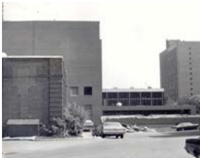
Macdonald (D) Building under construction during the building of the Nova Scotia Technical College's new administration complex, c1960-61
