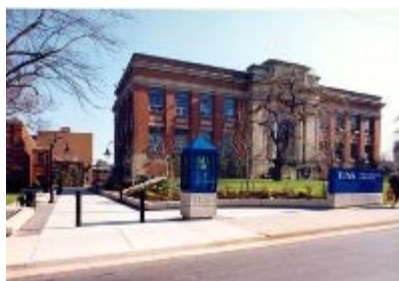
Architecture Building - Exterior - Front - 1, n.d.
