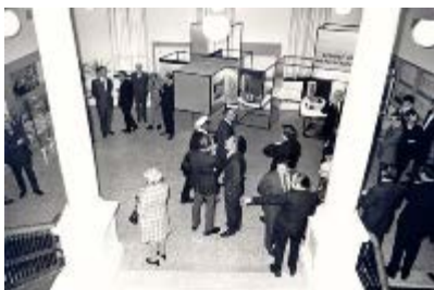
Official Opening of School of Architecture (H-Building) after Completion of Renovations - February 11, 1971
