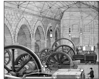
Interior cables housed (Shapiro)
