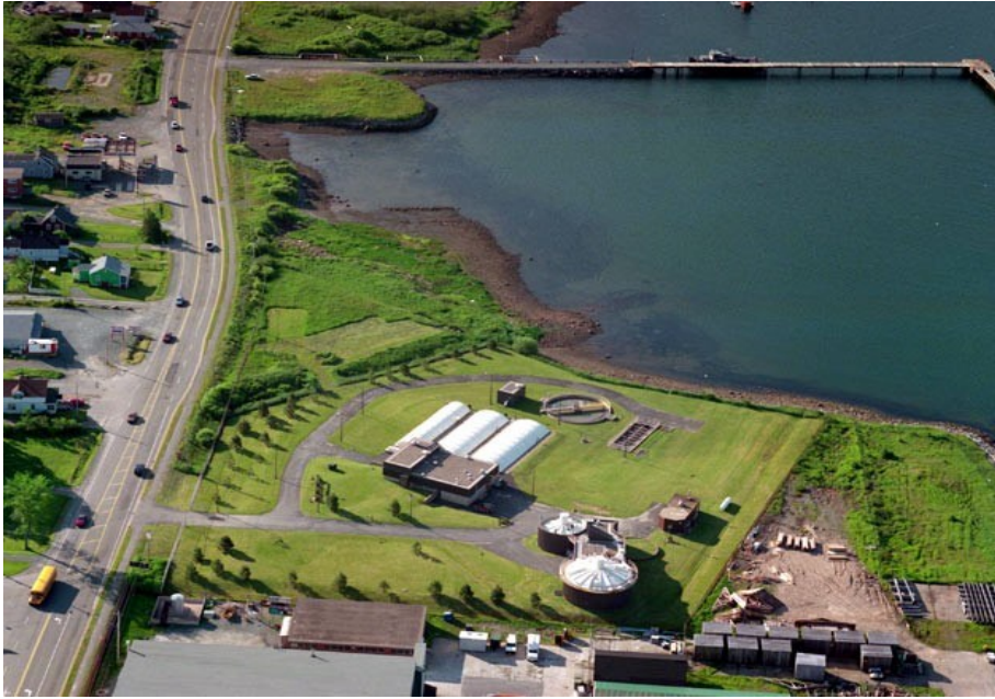
Figure 3-11 Top view of Eastern Passage WWTF (Halifax Water 2014)
