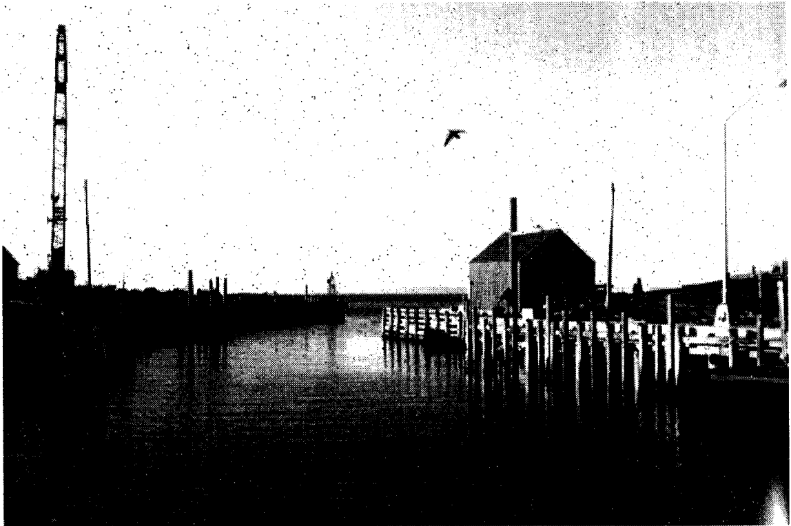
Figure 6-7: Hall's Harbor wharf in Nova Scotia
