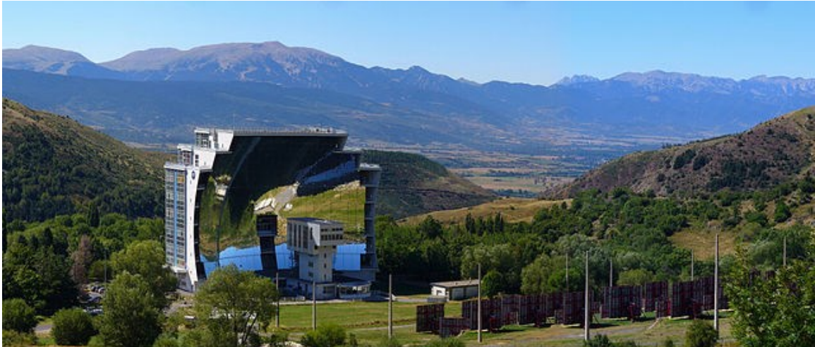
Figure 1-5. Odeillo Solar Furnace
