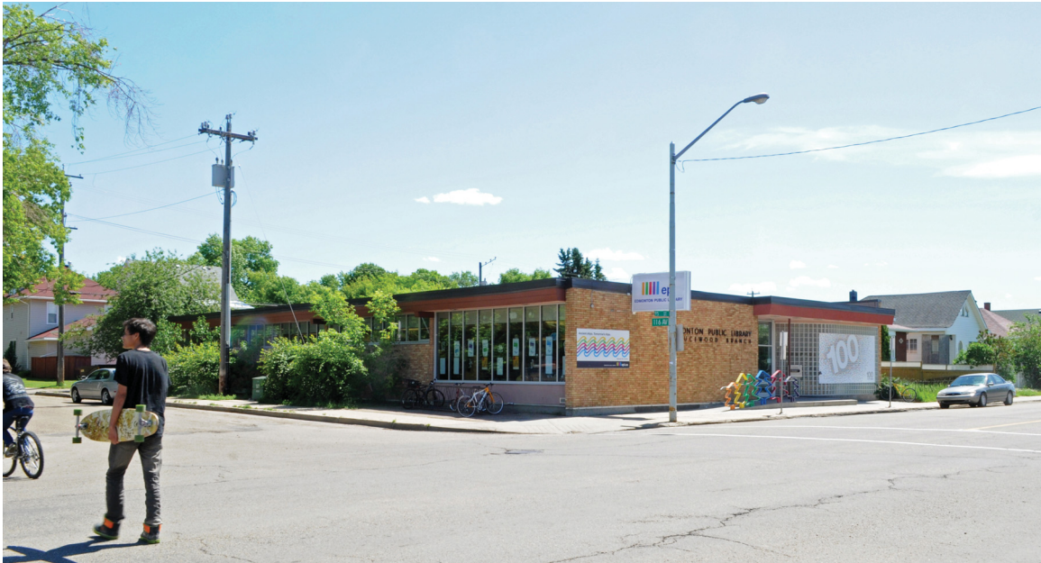
Existing Sprucewood branch, Edmonton, Alberta, 2013
