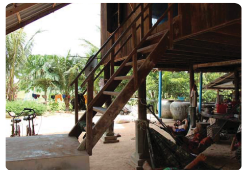
Main access (concrete block and wooden stairs)
