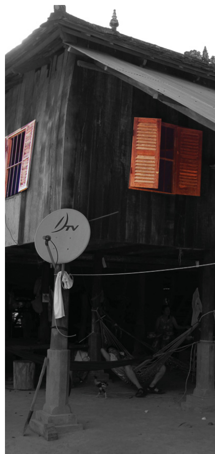
Windows with iron bars.
