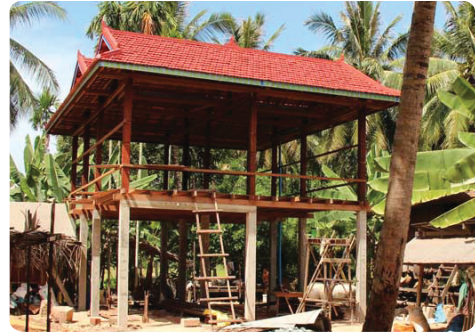
Construction of a traditional home
