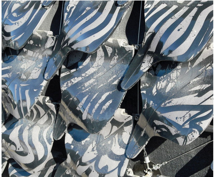
Photograph showing the glaze variation on Villa Nurbs; from Enric Ruiz Geli
