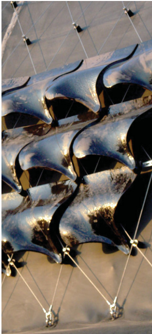
Photograph showing the connections of ceramic pieces in the Villa Nurbs; from Enric Ruiz Geli
