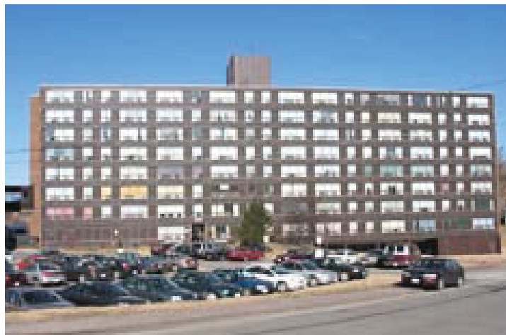
Exterior photo of Loch Lomond Villa / Nursing Home, St. John, NB from Cavare Home Care Ratings
