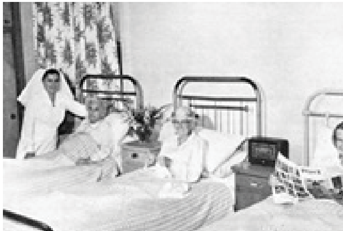
1940s rooms for the aged, Hammond Care Nursing Home, Sydney NSW from Hammond Care Nursing Home
