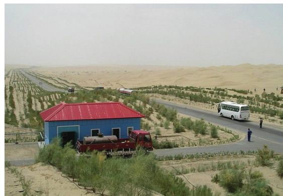
Takalamakan Desert pumping station (dmcooper_onechib, 2006)
