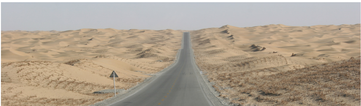
The cross desert highway, also known as the Tarim highway with desert vegetation planted on either side of the road helps reduce wind and soil erosion as well as restricting sand dunes from shifting onto the highway.
