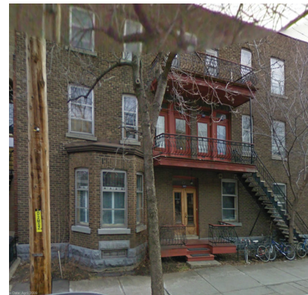
Fig. 61 Quintuplex on Mentana Street, Lower Plateau, Montreal, QC. (Image from Google streetview, 2009)
