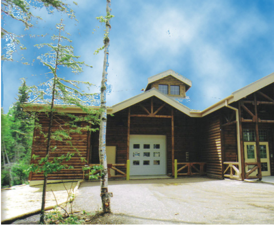
Wasagaming water treatment plant, 2004; from Bird Construction
