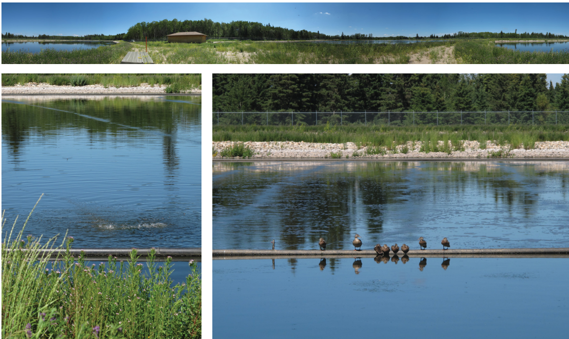
Wasagaming wastewater and sewage treatment facility, Wasagaming, Manitoba, 2012
