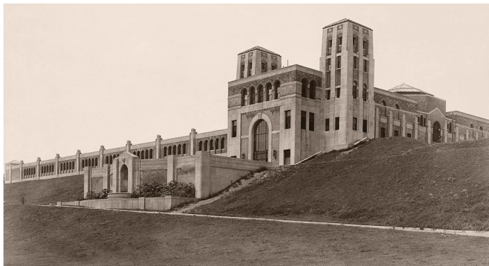
Photograph of the R. C. Harris Water Treatment Plant and park, Toronto, 1952; from Scarborough Historical Society
