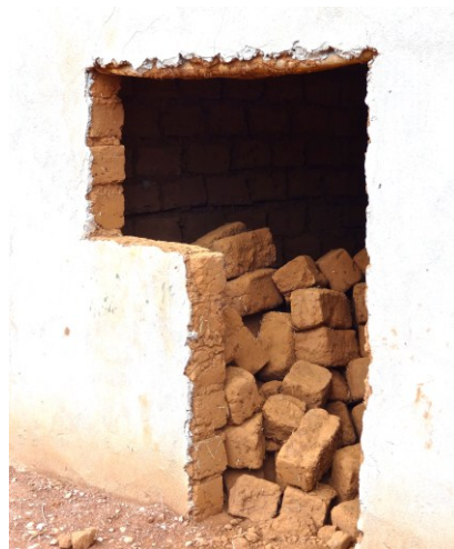
(Figure 7 – The bricks used in the construction process)
