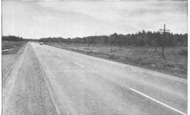
Soil-cement stabilization in New Brunswick Owned by: Province of New Brunswick. Minister of Public Works: Hon. A. F. Richard. Deputy Minister of Highways: W. T. Hargreaves.
