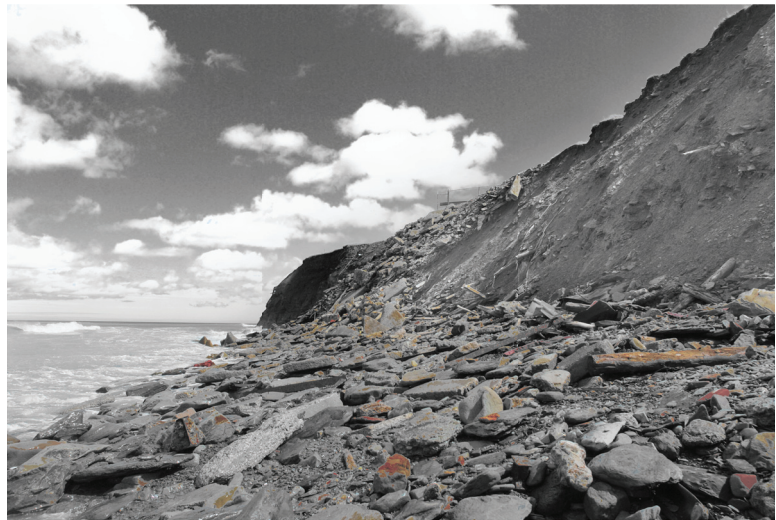
Looking east along the shore of the site of former Colliery 1B + 26.
