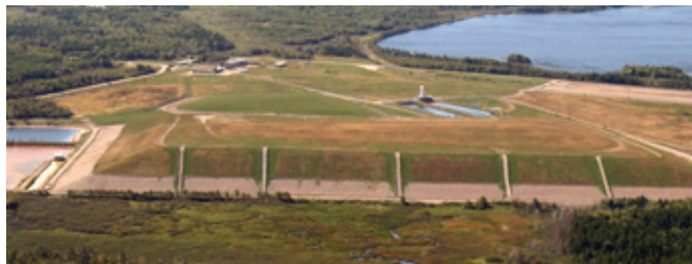
Victoria Junction - after remediation. Source: Public Works and Government Services Canada.
