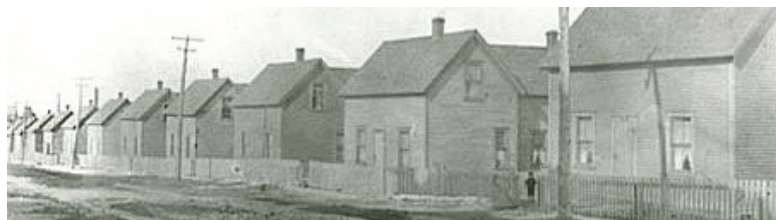
Housing provided by the mining company in Cape Breton. Source: Nova Scotia Archives, 1909.
