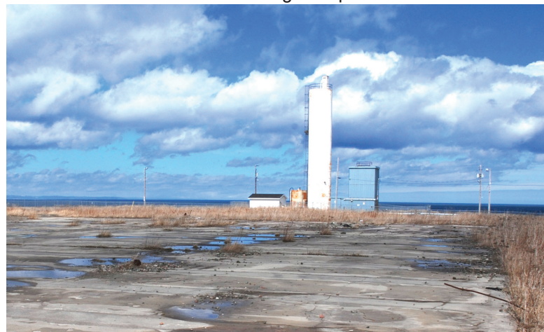
Former Site of Colliery 1B+26. Currently on the site is a tower for lime storage and minewater pumphouses.
