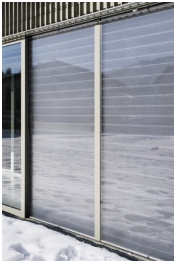
Figure 2-30: The GlassX, a smart window that uses phase change materials to extract solar energy and regulate room temperature. Image extracted from (Wilson, 2010)
