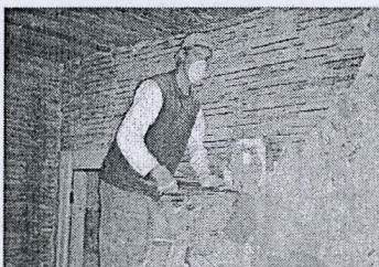
Demolition time! Photo: EAC
