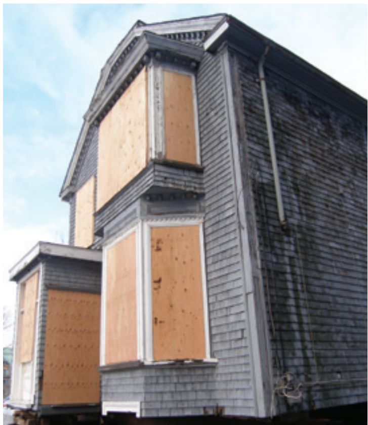
The Hollis Morris house awaits its new home.
