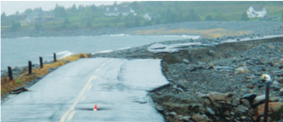
Causeway damage due to a storm surge after Tropical Storm Bill.
