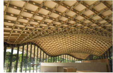
Interior of structure. Image from Harris, The Saville Garden Gridshell Design and Construction
