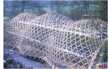
Finished structural from Harris, Downland Gridshell: An Innovation in Timber Design
