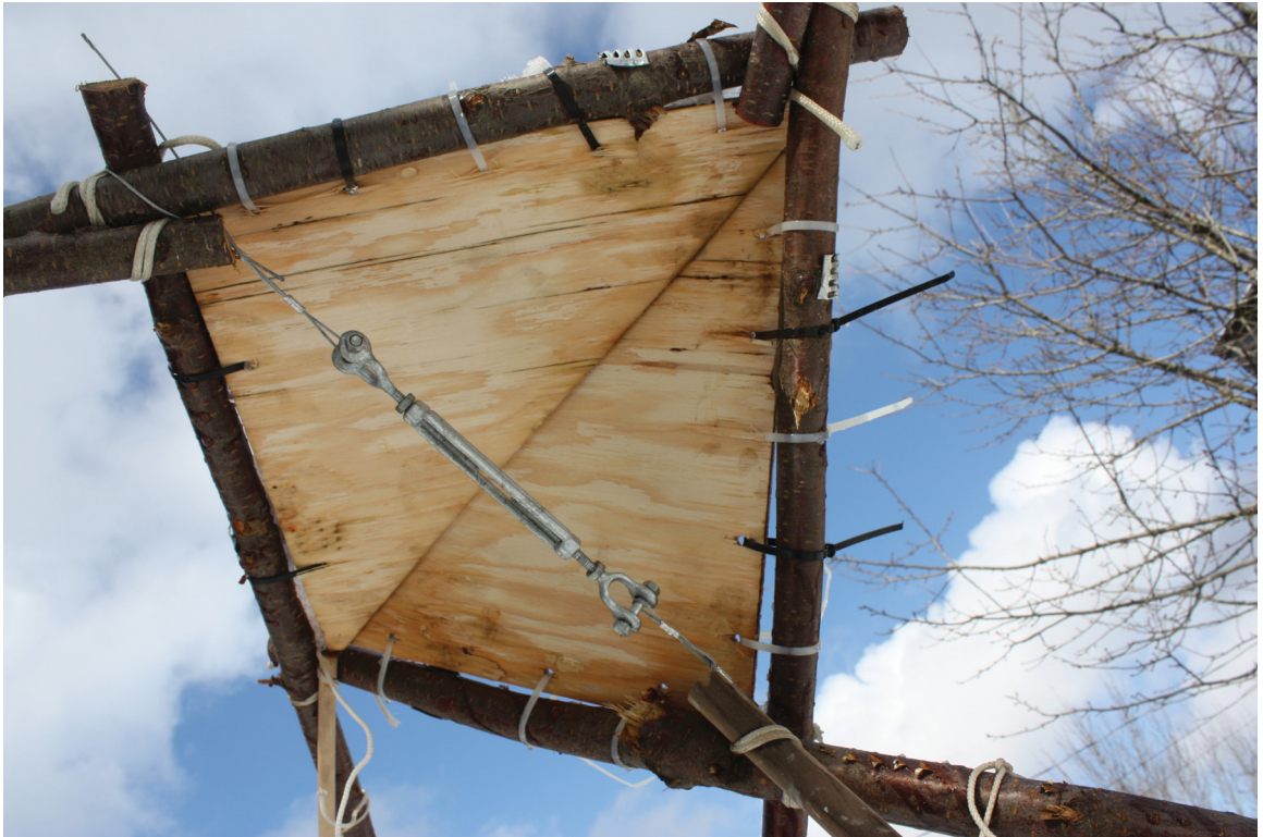
Final connection detail
