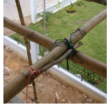
Scaffolding tie in context from C.A.S.T.
