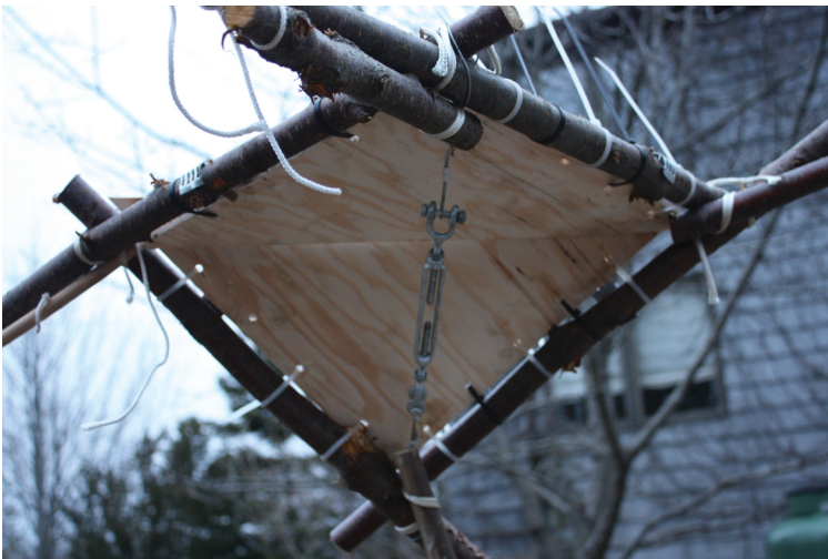
Underside of the connection shows the tension member pulling the system into tension
