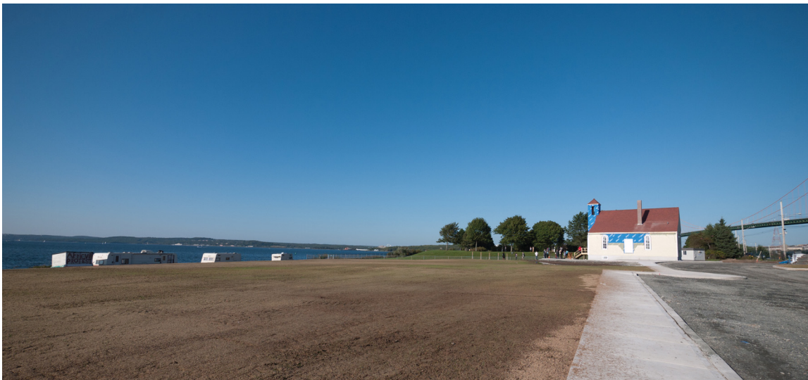
New replica church under construction in Africville. Eddie Carvery's Residence on left, 2011.
