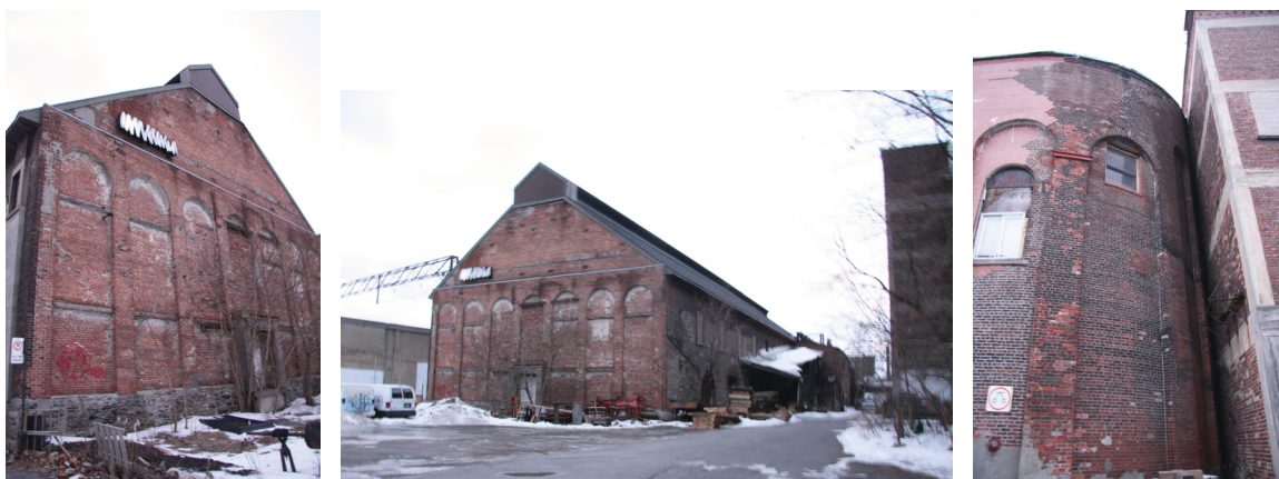
Photographs of the New City Gas complex in its actual condition.
