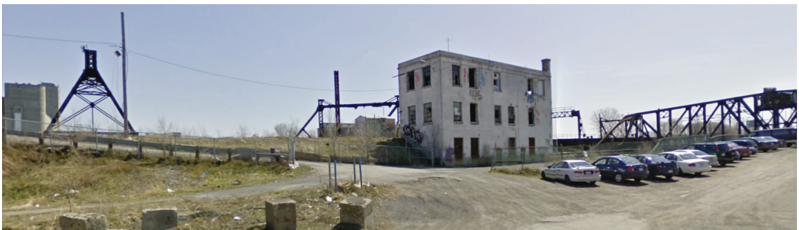
Photographs of the CN Wellington building.
