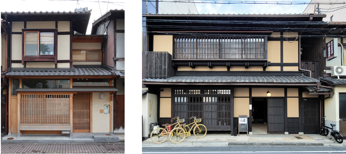
Examples of machiya facades from fieldwork conducted in Kyoto. The left machiya is standard width while the machiya on the right is doubled in width.
