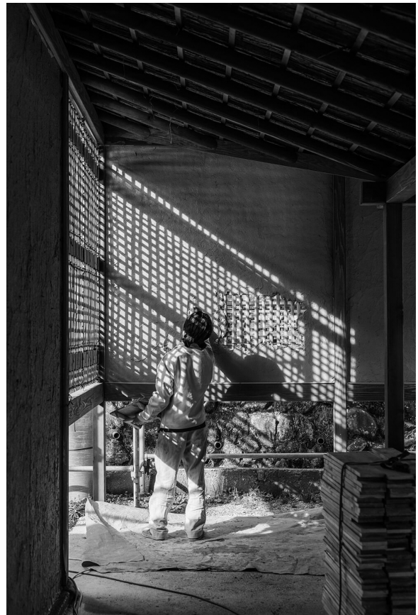
A craftsman applying plaster (Anami and Nagao 2023)
