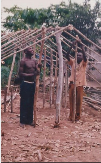
Figure 41: Inhabitants of an “Ujamaa” village building their homes with local materials and traditional forms. (Darby 2015)
