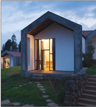
Figure 28: The Butaro Doctors' Housing completed through a holistic design built using locally sourced materials such as volcanic rock. Photograph by Iwan Baan (MASS Design Group n.d.-c.)
