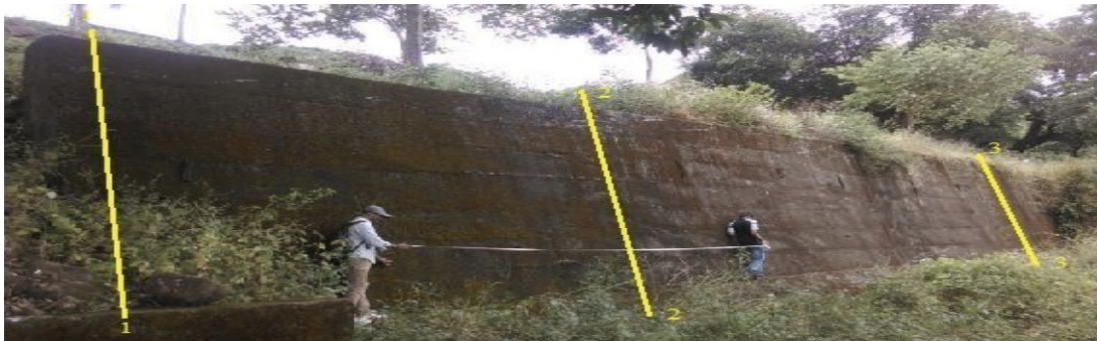
Fig 2.2 Existing Retaining wall at Dewarwadi (Vijayakumar et al., 2015)
