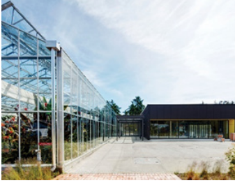
Sechelt Water Resource Centre (PUBLIC Architecture + Communication 2015).
