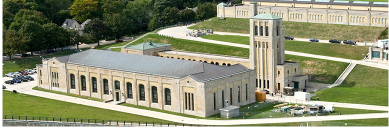
R. C. Harris Water Treatment Plant (City of Toronto n.d.)
