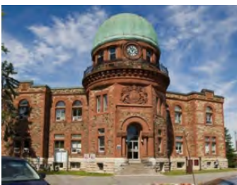
Photograph of the Dominion Observatory building at the Central Experimental Farm (McGrath 2022).
