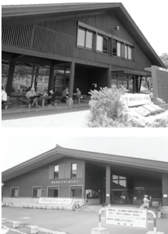
Figure 17-18: Engineered volcanic roofs on refuge facilities (Yamada et al. 2020)
