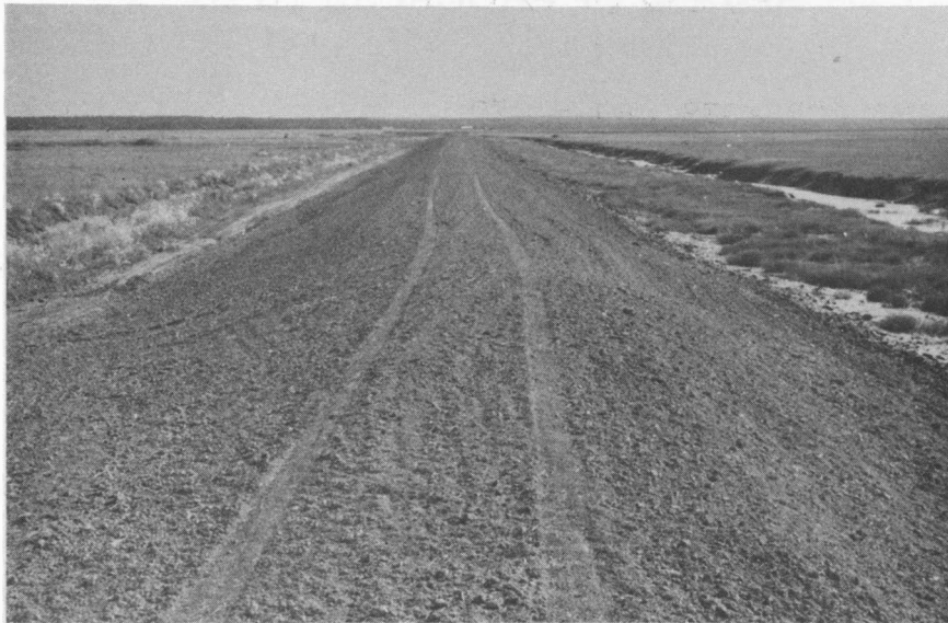
Figure 5 - Minudie Marsh, Cumberland County, N.S. Typical section of new dyke with seeding just completed. Borrow pit to the right.
