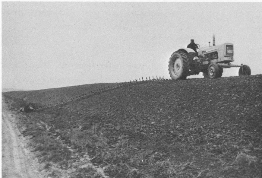
Figure 5 - Minudie Marsh, Cumberland County, N.S. Typical section of new dyke with seeding just completed. Borrow pit to the right.
