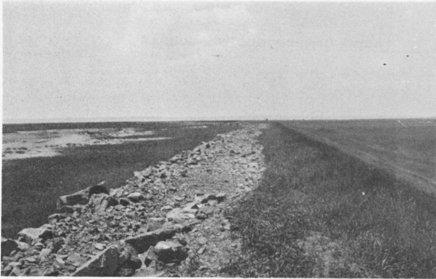
Figure 3 - John Lusby Marsh, Cumberland County, N.S. Standard rock facing on tidal side of dyke. Rock protects dyke from wave action and tidal currents.
