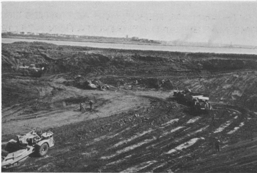
Figure 1 - Petitcodiac River Dam, Westmorland County, N.B. Start of excavation for the re-inforced concrete control structures, early in 1966.
