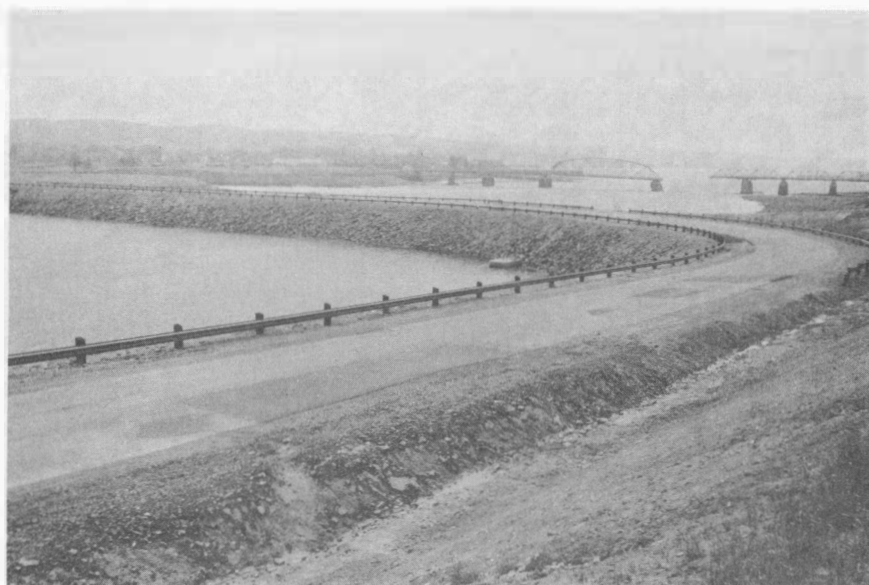
Figure 2 – Annapolis River Dam – Looking downstream across the rock-fill causeway toward the old Granville Ferry bridge. This main highway crossing replaces the old bridge which failed just prior to completion of the causeway.
