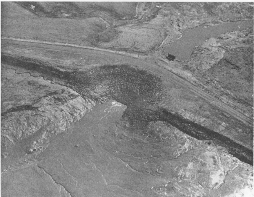
Figure 2.-- Aboiteau #1, Wellington Marsh, Kings Co., N.S. Asbestos bonded steel corrugated pipes were threaded through the old sluice and extended downstream to allow placement of a stable rock face. New inlet cribs and emergency shut-off gates were also constructed.
