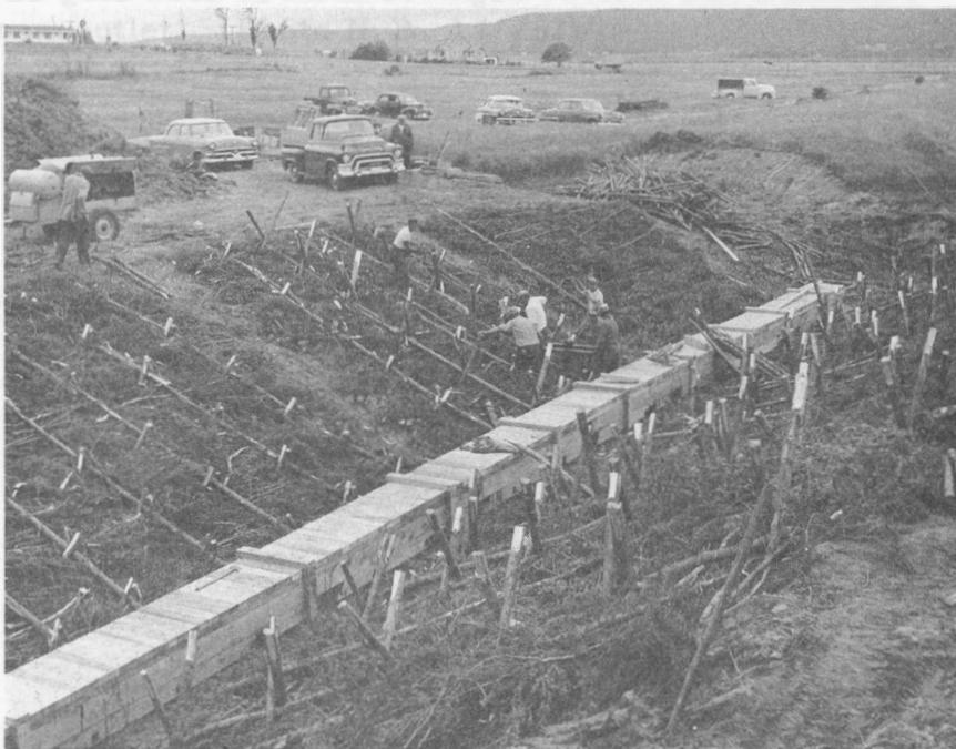
Fig. 10 - Abt. #1 on Allan River Marsh, Anna. Co., N.S., under construction. The sluice has been set on its bed, and brushing of the aboiteau fill is in progress. Brushing, as shown here, is done between every 2 ft. layer of fill. (Photo N.S. 30//10)
