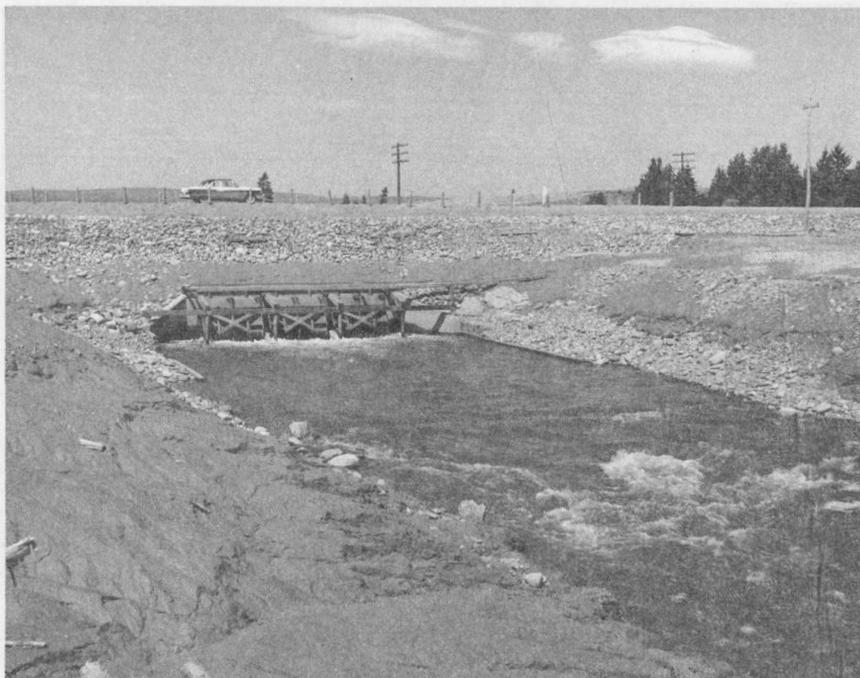
Fig. 14 - A general view of the completed works on the Isgonish River, Col. Co. , N.S. This large sluice of reinforced concrete, is under the new Trans-Canada Highwa and replaces a single-lane bridge which was located off the right of the photo. (Photo 15-025)
