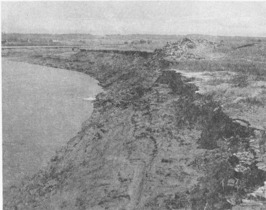
Fig. 7 - Bank erosion on Memramcook West Marsh, West. Co. , N.B. The Memramcook River has worn away the outside berm, until only 15 ft. remains between the bank and the toe of the dyke, which is in danger of undercutting. The pile of rock indicates that protective works are in progress. (Photo 21-037)
