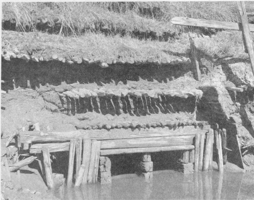
Fig. 13 - The inlet end of Abt. #3, Seaman Marsh, Cumb. Co. , N.S. The condition of this aboiteau is typical of many old aboiteaux which have fallen into a state of disrepair through lack of maintainance. Note the fill washed out from between the layers of brush. (Photo N.S. 55//3)
