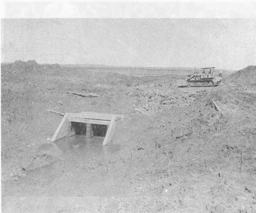
Fig. 2 - The inlet end of an aboiteau under construction
