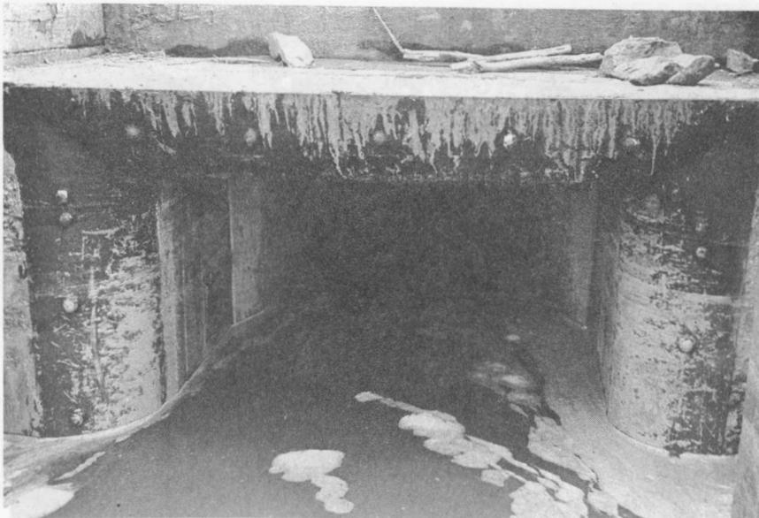
Fig. 9 - A rounded inlet to the sluice through Abt. #5, Glenholme Marsh, Col. Co., N.S. The quarter-round steel section is lag screwed to the ends of the timbers, and filled with concrete. There is a noticeable improvement in flow through the sluice as a result. (Photo 64-023).
