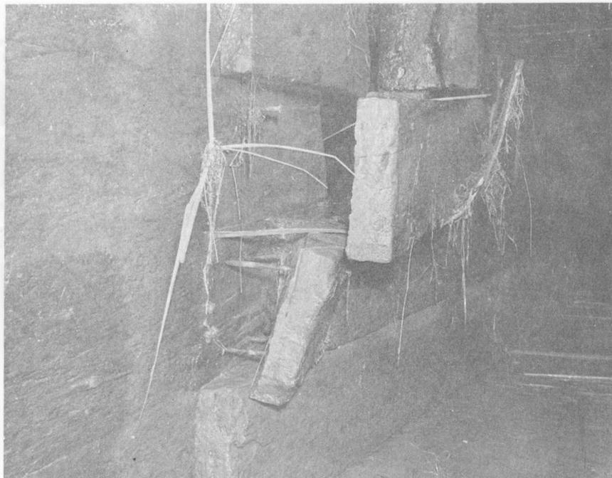
Fig. 3 - Inside the barrel of Abt. # 1, Wellington Marsh, Kings Co., N.S., showing the division wall timbers badly broken up. This old sluice had previously been temporarily repaired by the M. M. R. A. until such time as permanent repairs could be undertaken. (Photo 56-017)
