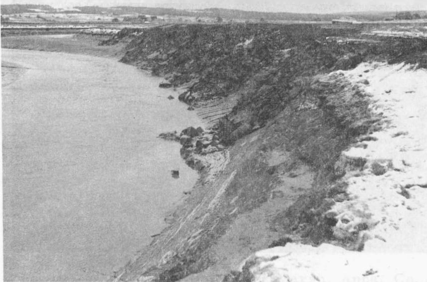
Fig. 8 - The same view as in the above photograph; after heavy rock has been placed over the bank in a series of piers. This method proved to be the most permanent protection against undercutting. (Photo 21-054).
