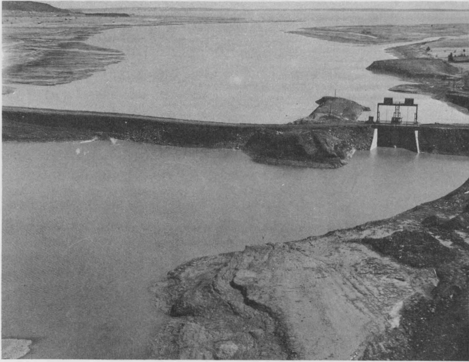
The Shepody River Dam, Albert Co., N.B.—Rock fill and fresh water discharge facilities prior to the fill being brought to final grade and cross-section. This is the upstream side of the structure as one looks towards the mouth of the Shepody River. The marsh shown in the upper right corner is protected by dyke which connects with the left or north end of the dam. The balance of the marsh protected lies upstream of this structure.
