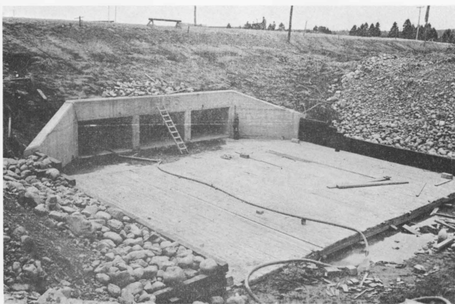
The upstream side of the Isgonish bridge-aboiteau in the spring of 1955. The three sluices are each 6' x 10'. Rock will also be dumped at the upper end of the plank spillway. (Photo N.S. 15/105).
