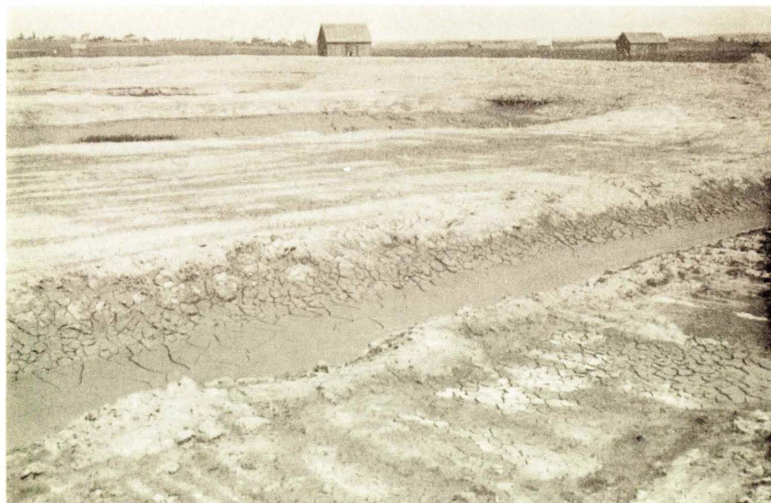
Fig. 16 - Project N. S. 42, Amherst Point Marsh, N. S. This is a view of the completed structure shown under erection in Figures 13 and 14.
