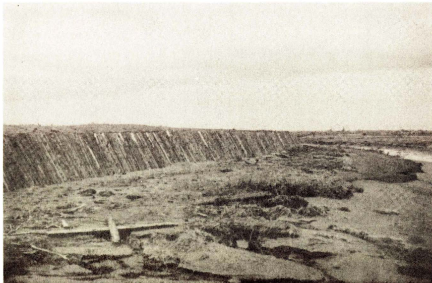
Fig. 2 - Project N. B. 5, Westcock Marsh, N. B. A section of slab facing erected to prevent the dyke against severe wave action.
