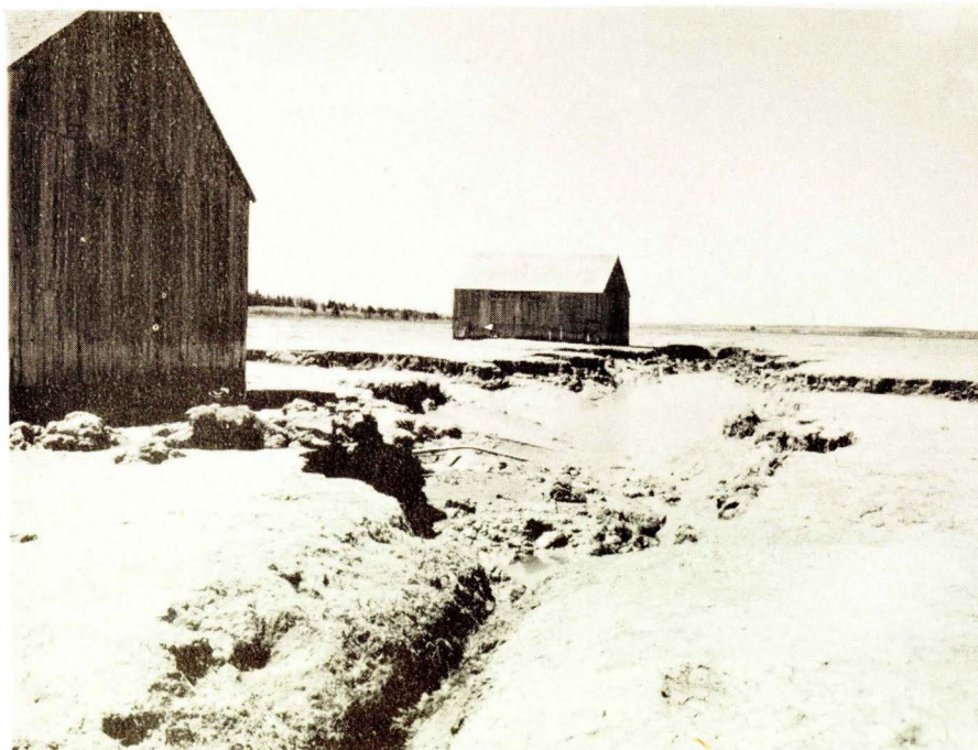
Fig. 26 - Project N. S. 53, John Lusby Marsh, N. S. This is a view of damage which occurs to land after the protective structures have been allowed to deteriorate and tide water is permitted to flood the area. The damage is caused by the tide water flowing off the marsh.
